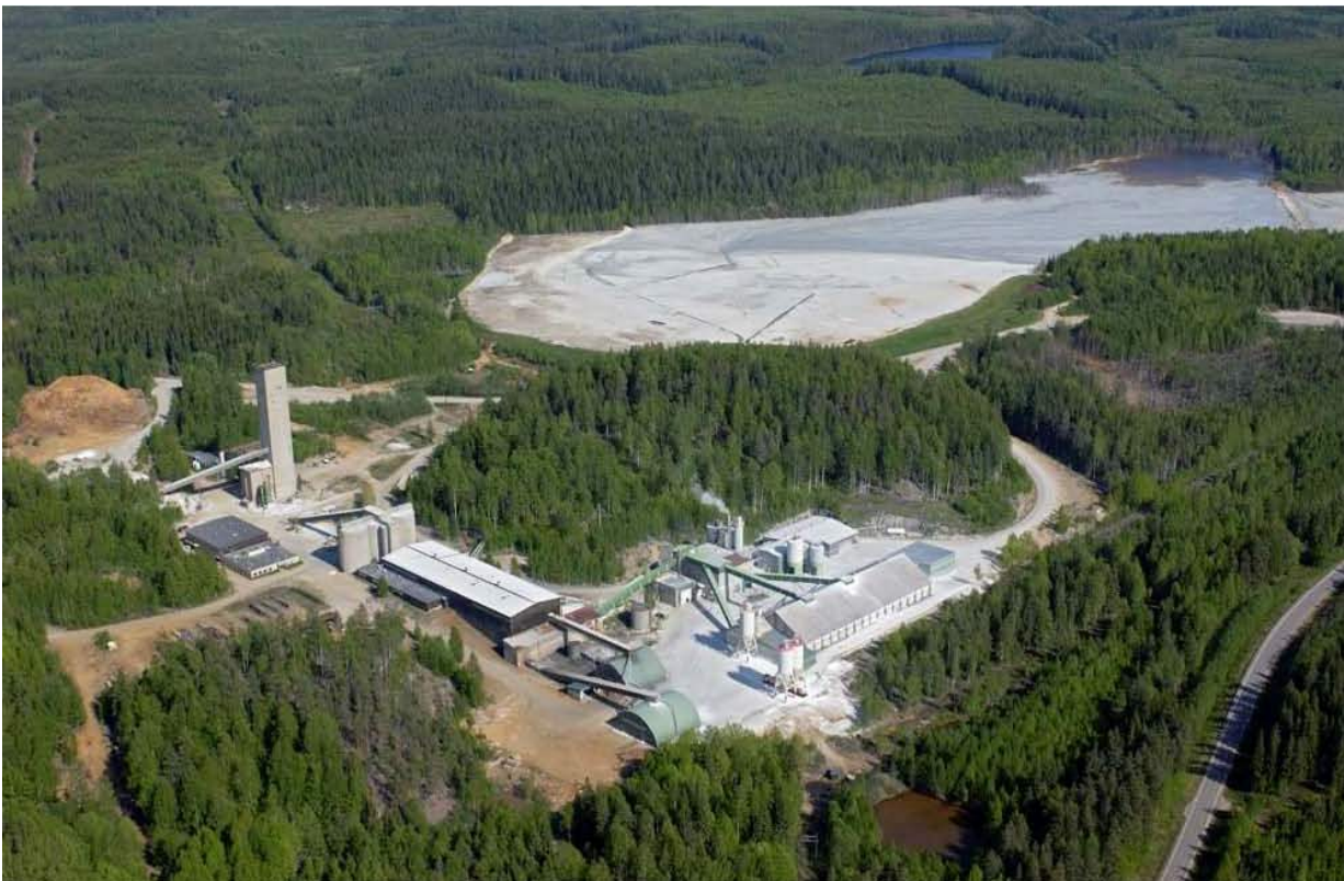
Luikonlahti Processing Plant and Tailings Dam
