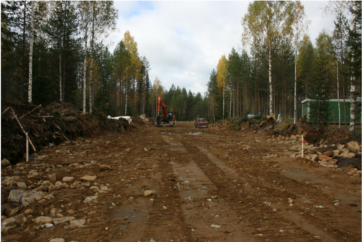
Access road at the Kylylahti minesite
