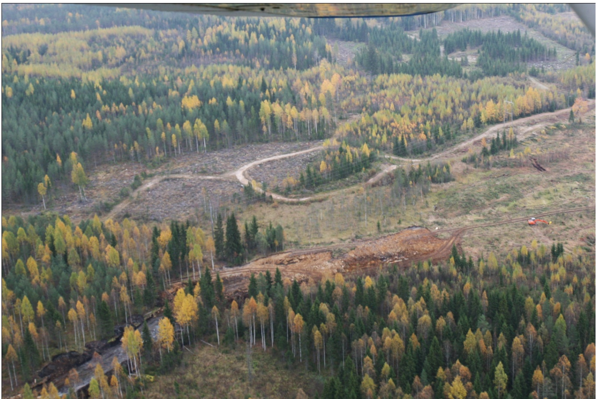
Access road and office site Copyright Markku Mutanen
