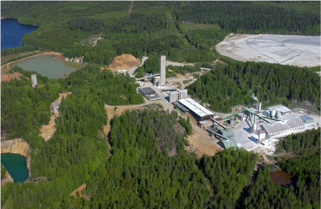
Figure 1: Aerial View of Luikonlahti Processing Plant
