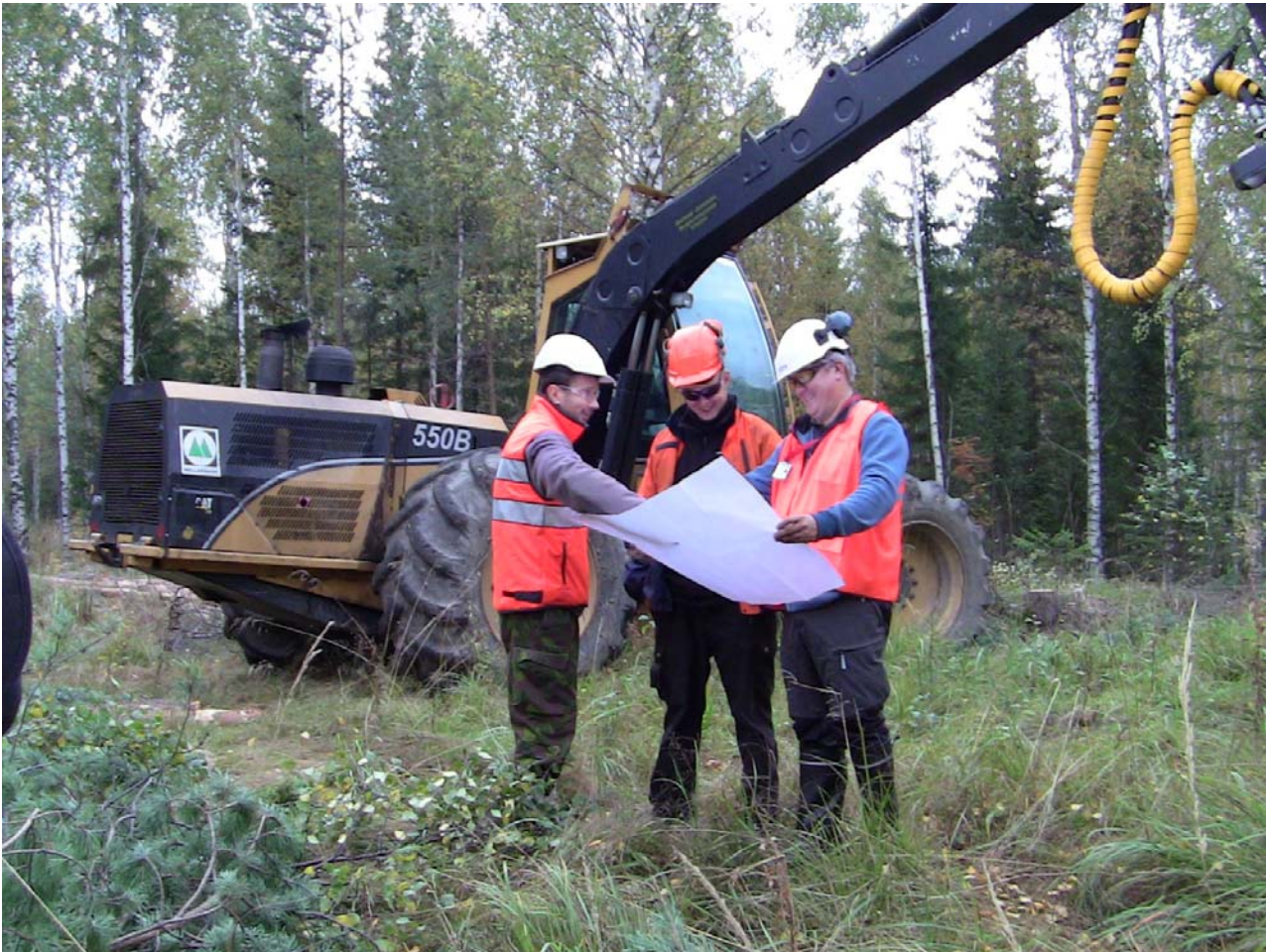
Figure 1: Commencement of site clearing at the Kylylahti mine site. Mine Manager Seppo Tuovinen on the left
