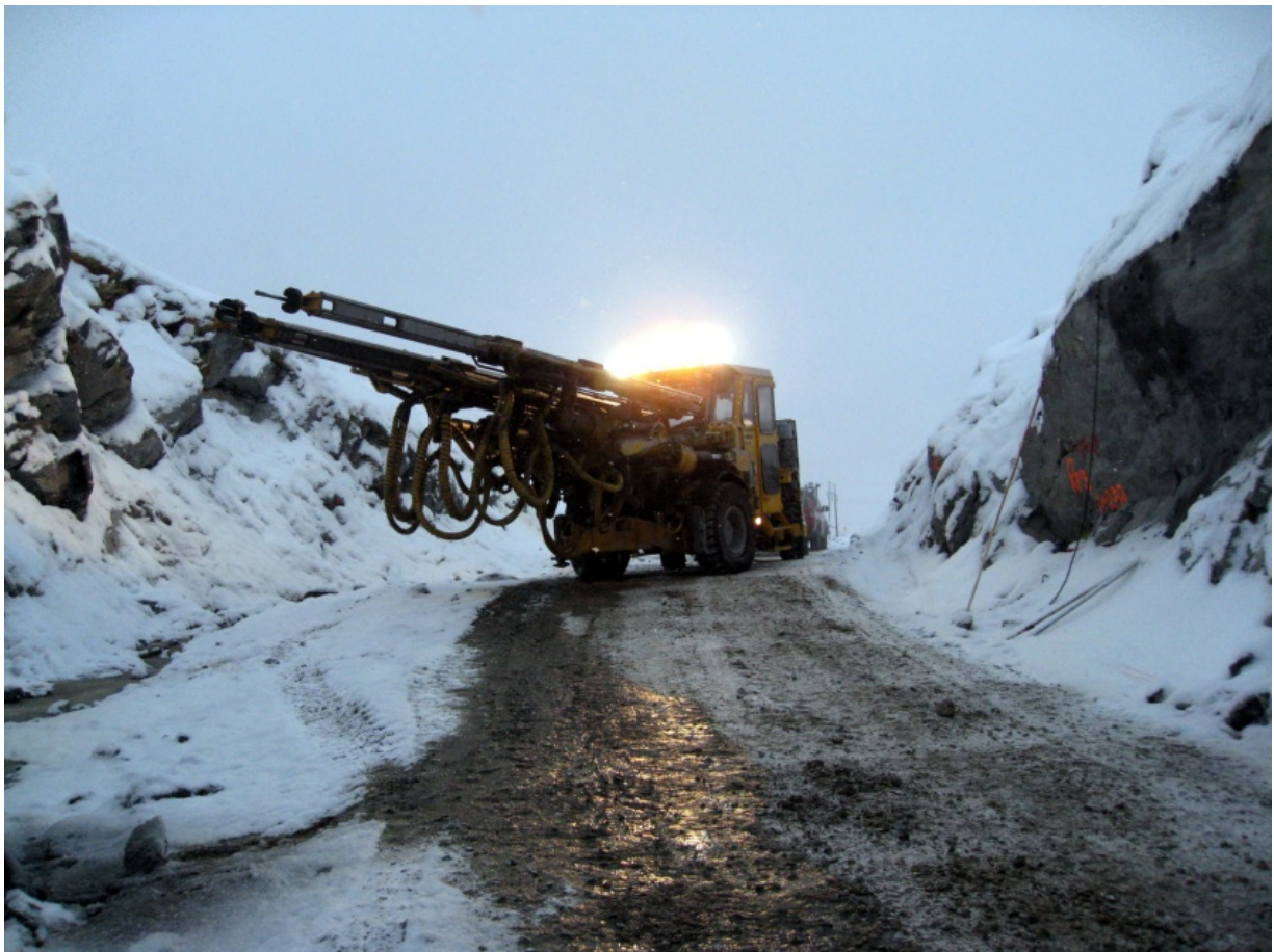
Jumbo (drilling machine) at the Kylylahti mine
