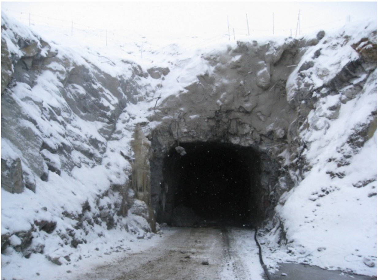
Kylylahti mine portal
