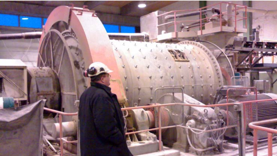
Primary Grinding Mill
