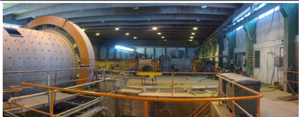
Figure 1: SAG Mill and flotation cell in the background at the Luikonlahti processing plant
