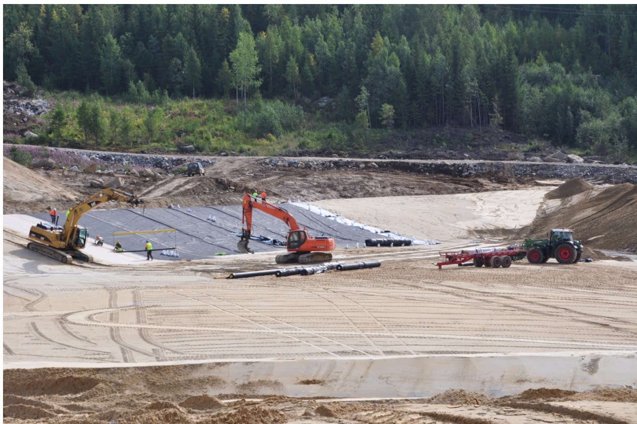
Installing lining to new concentrate storage dam at the Luikonlahti mill
