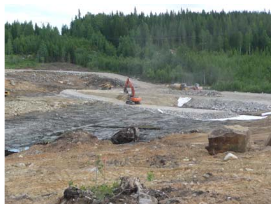
Earthworks at concentrate storage dam
