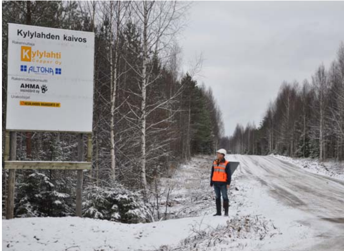
Access road to the Kylylahti mine site dewatering
